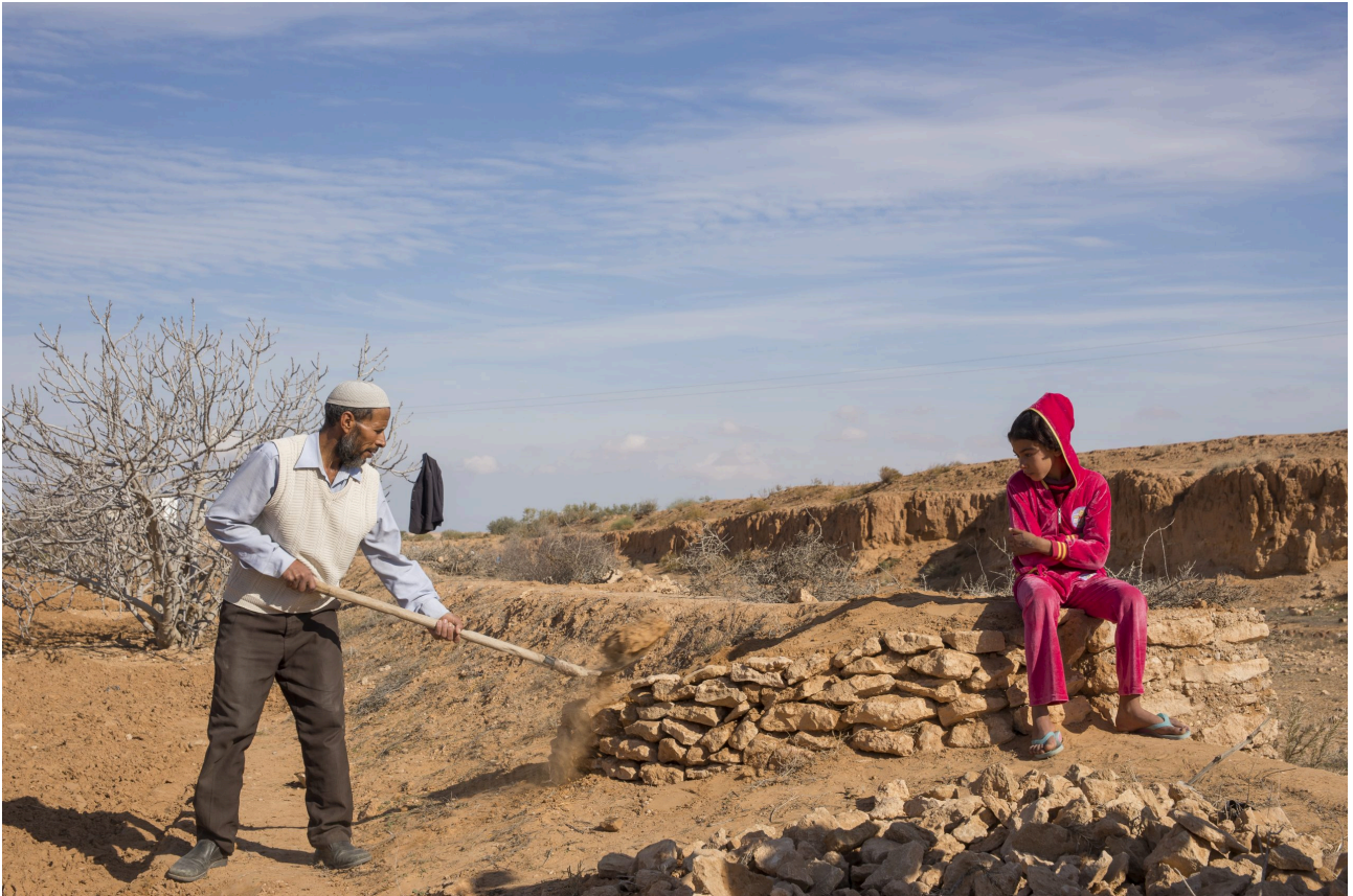
A farmer in Tunisia uses stones to build a jessour for water harvesting
